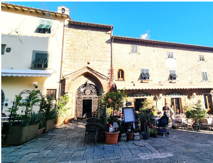
Figure 9 – Tavarnelli Tower with the Chapel of the Square
